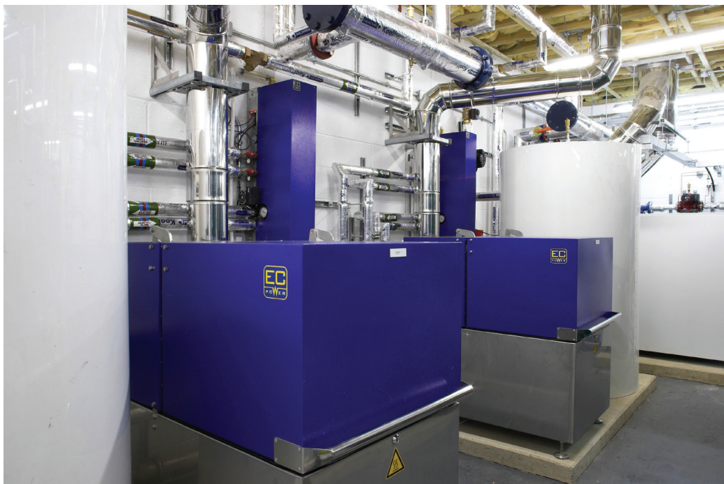
Figure 1: Installation of two LoadTracker CHP systems.
